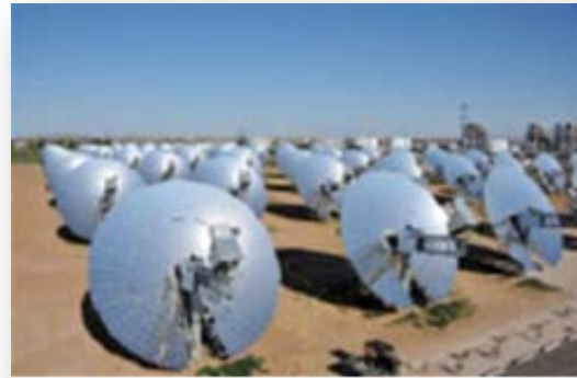
Fig4. Solar plant with SCADA
